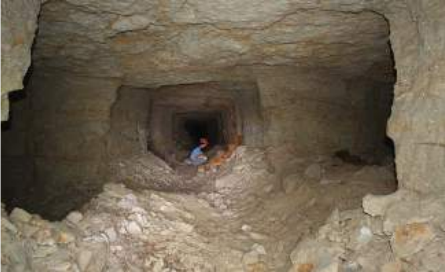
Figure 4. Looking along the axial aisle of the Dog Catacomb. The effects of scabbing can be seen at the foot of the walls (photograph: P.T. Nicholson).
