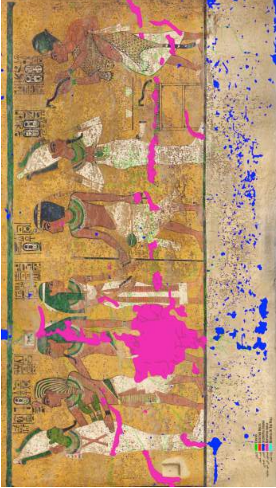
Fig. 27. Burial Chamber (J), KV 62: north wall, showing repainted areas (in pink), incidental damage (blue), cracks (green) and injection holes for consolidants (red) ( http://www.highres.factum-arte.org/Tutankhamun/ , copyright © Factum Arte/Ministry of Antiquities, Egypt)
