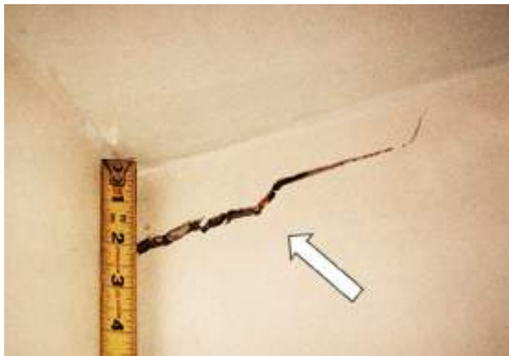
Fig. 17. Above: Burial Chamber (J), KV 62: north wall, surface relief (positive), showing diagonal separation in plastered surface. Below: Identical type of fissure as seen in a modern partition wall (Above: http://www.highres.factum-arte.org/Tutankhamun/ , detail, with additions, copyright © Factum Arte/Ministry of State for Antiquities and Heritage, Egypt, detail. Below: after http://inspectapedia.com/vision/SinkingHouse109DJFs.jpg , manipulated, with additions, copyright © InspectAPedia.com 2010)
