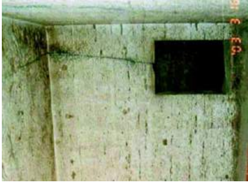
Fig. 9. Vertical faulting above door lintels in (left) KV 62 (Tutankhamun – entrance to the Treasury, Ja) and (right) WV 22 (Amenhotep III – entrance to side room Jbb) (Left: http://www.highres.factum-arte.org/Tutankhamun/ , copyright © Factum Arte/Ministry of State for Antiquities and Heritage, Egypt. Right: after Yoshimura and Kondo 2004, 92, fig. 11, copyright © Institute of Egyptology, Waseda University/UNESCO)
