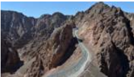
Fig.9 Road cut in a hard rock site [17].
