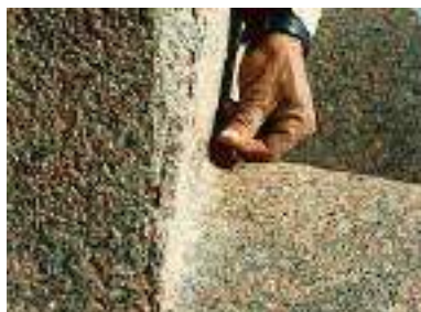
Fig.3 Filleting corners of granite mating surfaces [11].
