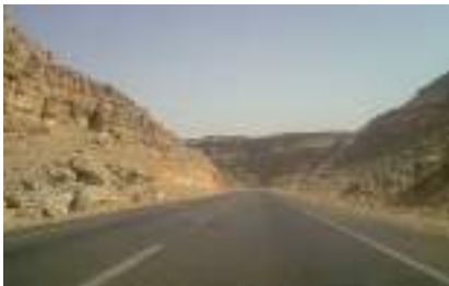
Fig.8 Highway cut in a limestone site [16].
