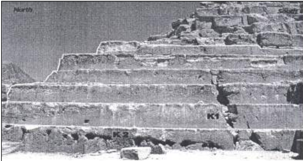
Fig. 7 Khephren Pyramid. View of the northern part of the W face. The visible part of the original hill (delimited by the white line) shows horizontal steps without horizontal or vertical block breaks (K1: Karst natural fracture; K2: discontinuities showing advanced dissolution processes along the strata surface). 9
